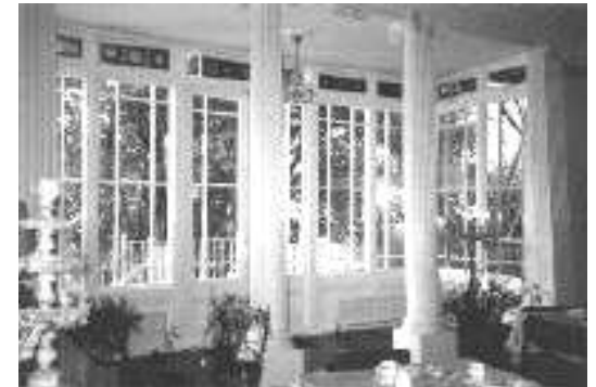
The Music Room window, installed in 2003
